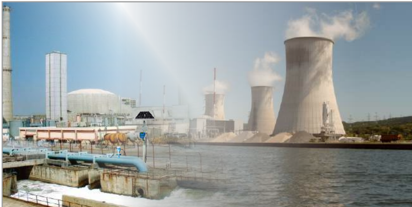
Use of MVBAR In Water Intake Flow & Pressure Measurements in Nuclear Power Plant
